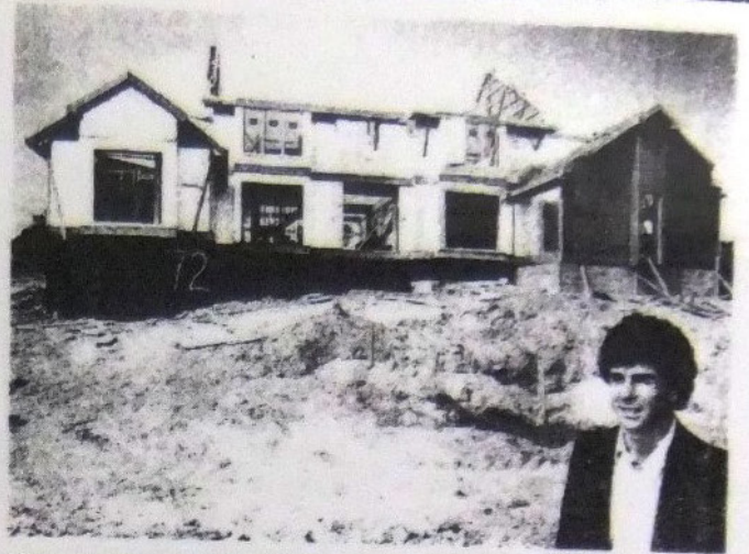
David Steuer in front of $395,000 house he designed
